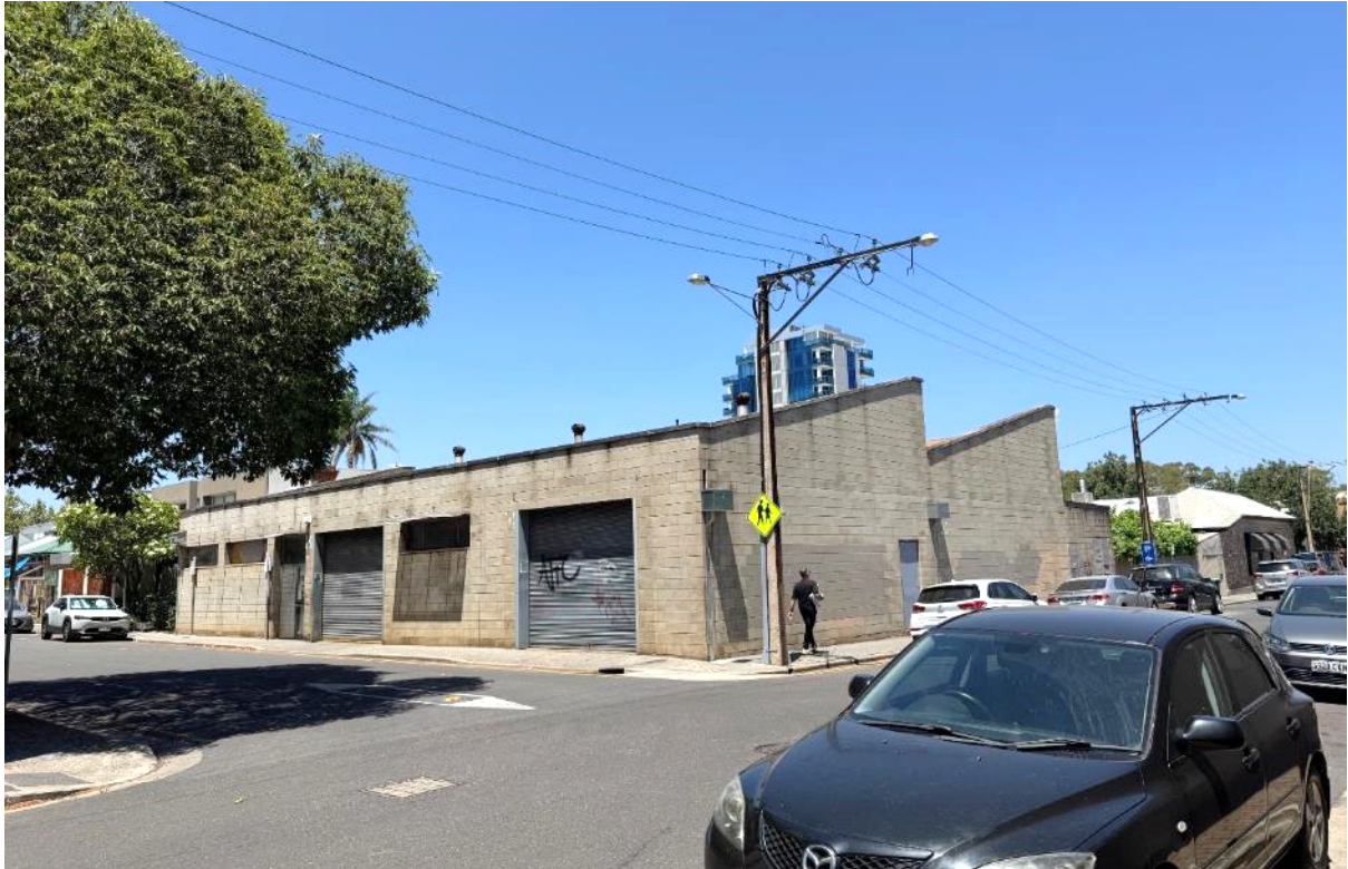
Figure 3.2 – Subject site from Cardwell Street
